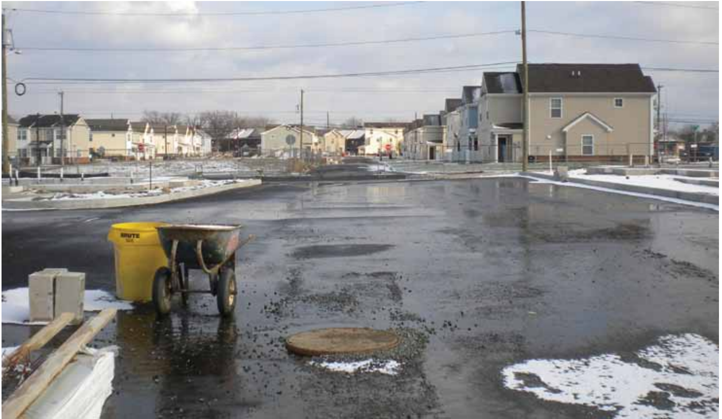
Roosevelt Manor with underground stormwater detention system below the street.
