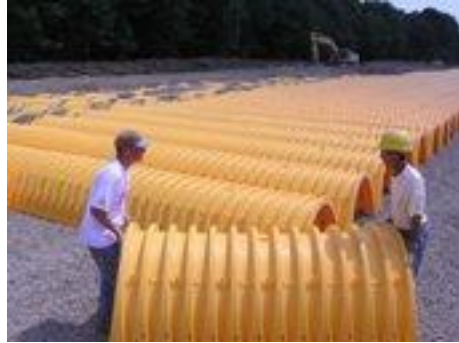
Figure 7. Installation of Corrugated Arch System (Stormtech®)
