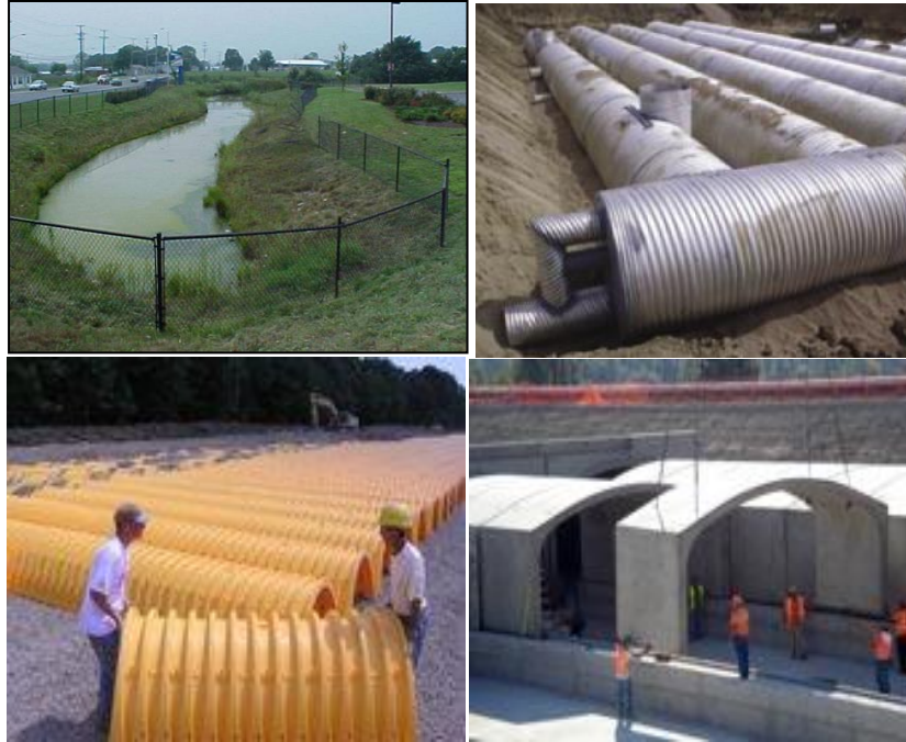
Figure 4 (a) Retention Pond (ACF Environmental) , (b) Corrugated Metal Pipe (Contech) , (c) Arch Chambers (Stormtech®) , (d) Conspan® (Contech)
