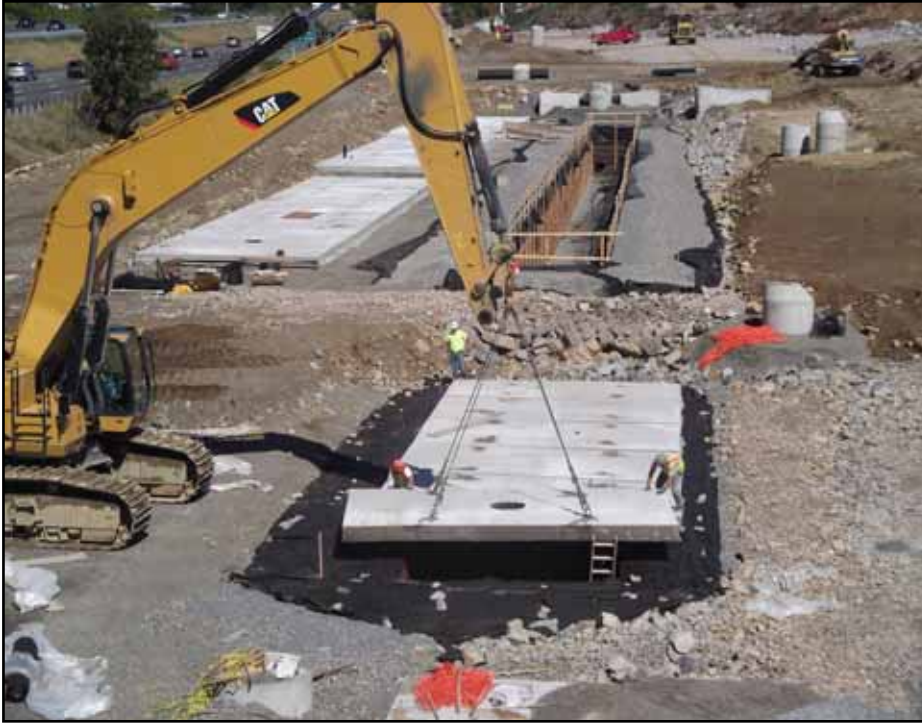
Roof slab installation.
